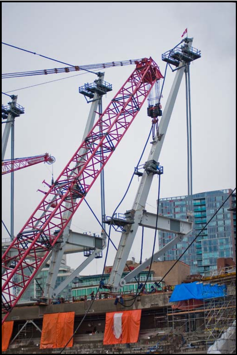
BC Place Construction
